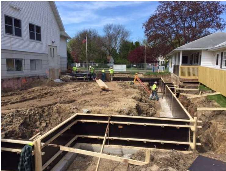
Footings and foundations at the addition are being formed up. Findorff Iron workers are on site tying up rebar so the carpenters can finish the other side of the foundation wall forms.
