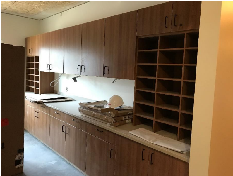
1 st floor copy/work room casework is installed.
